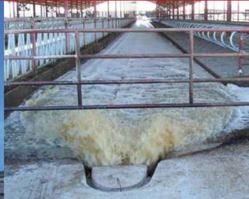
Above Ground Flush Valve with Two Floating Pumps
