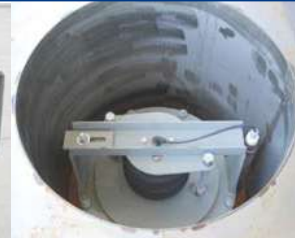
Air Operated Flush / Valve Insert
